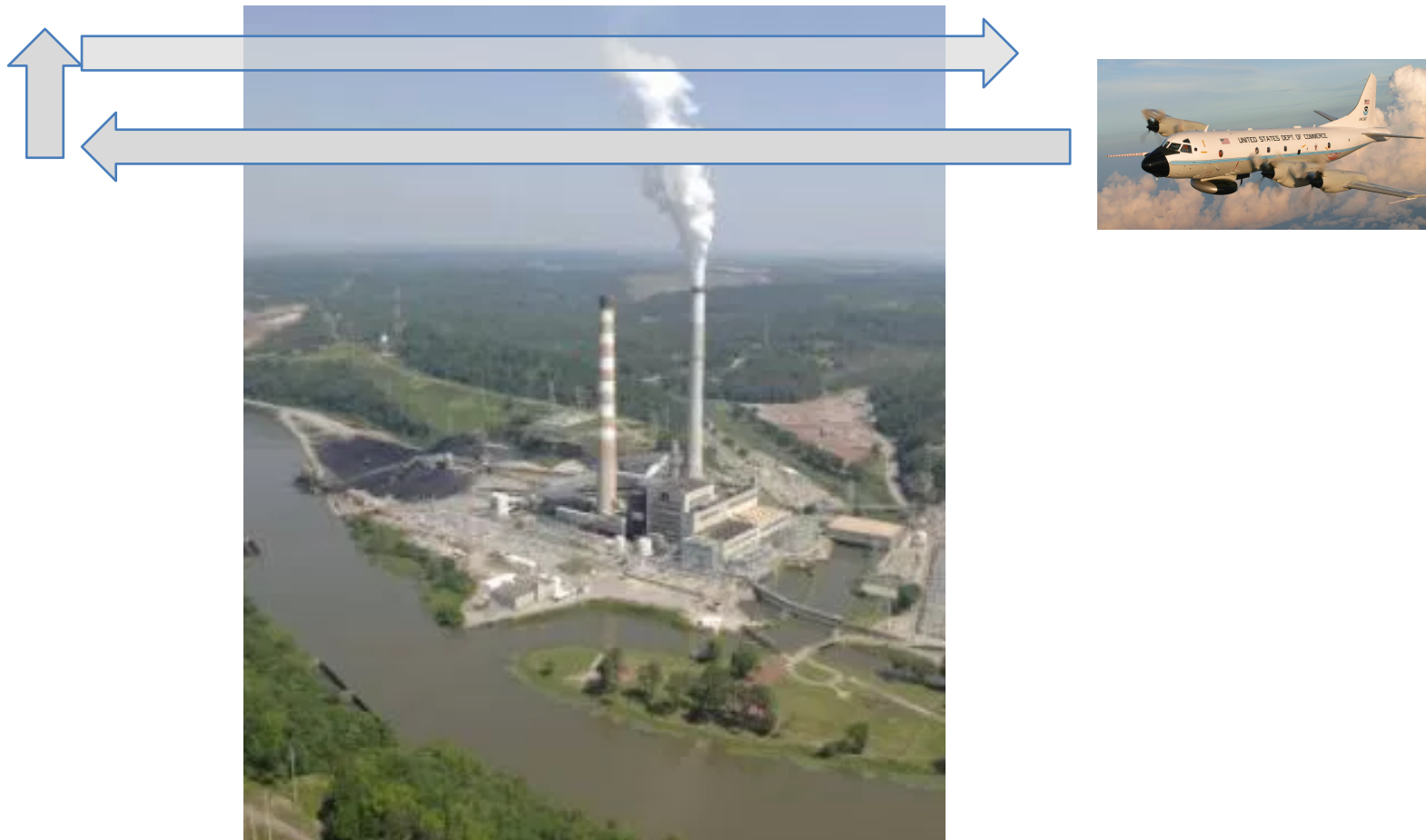
Gorgas steam plant, Parrish, Alabama
